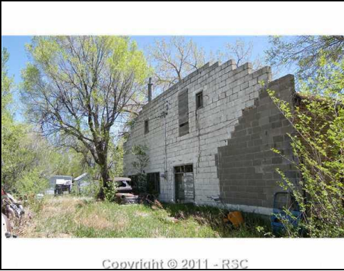
Copyright © 2011 - RSC Exterior Back Rear of Garage
